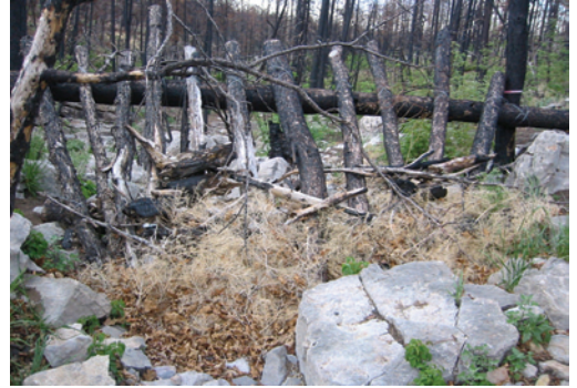
Image above shows debris buildup caught by trash rack built by local youth in the Manzano Mountain area.
